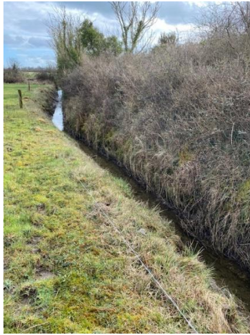
Field Drain near Turbine 2
