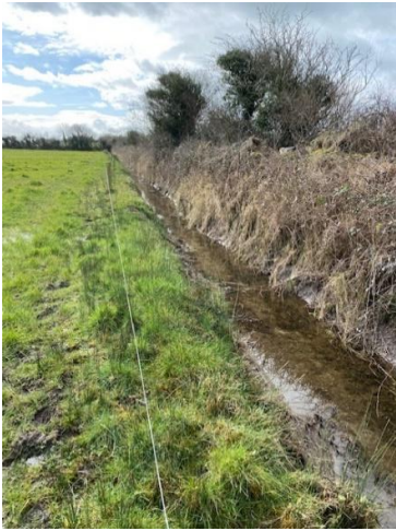
Field drain near Turbine 4
